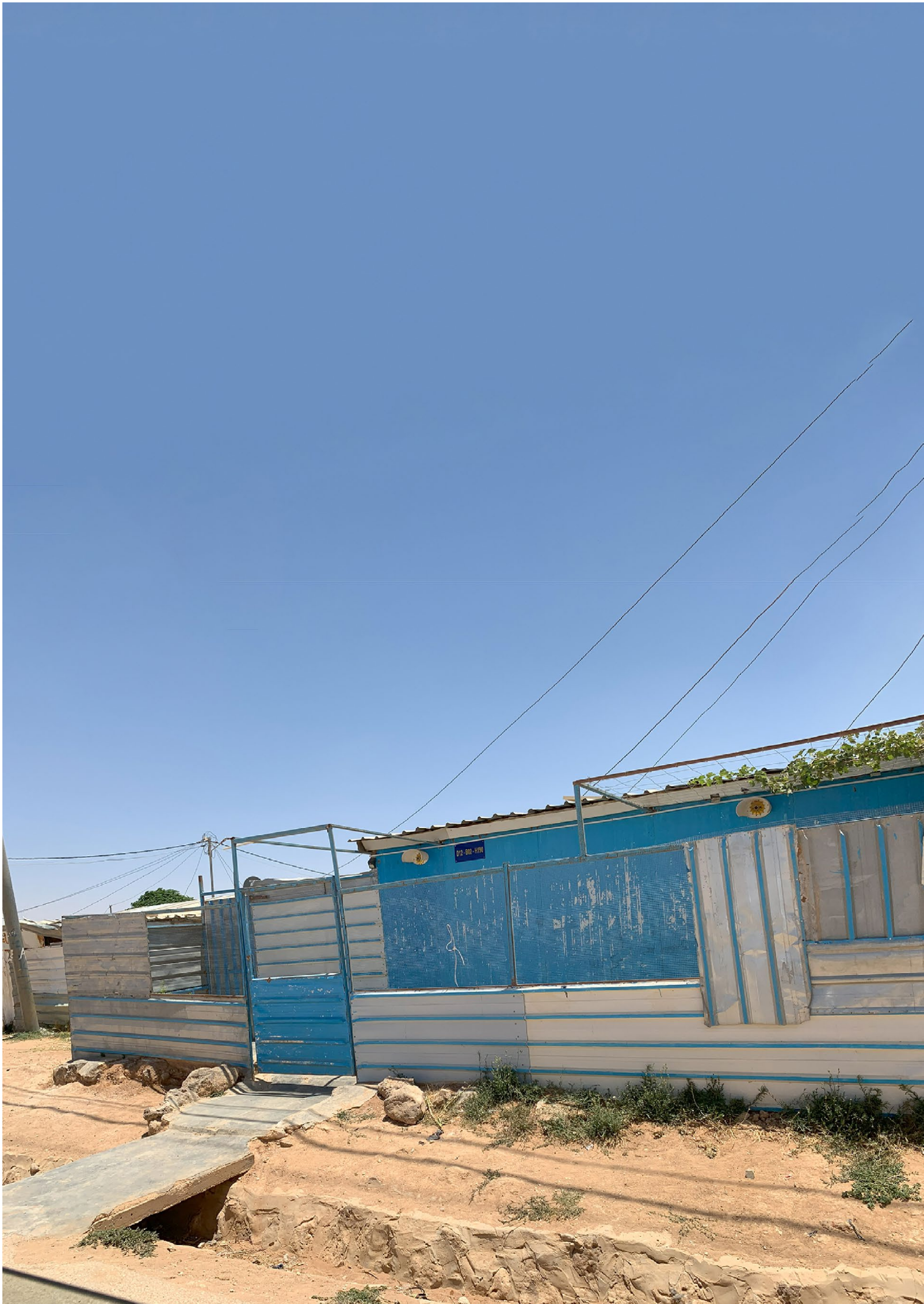
Figure 09. Exterior of a home created by joining several shelter units and adding a porch.
