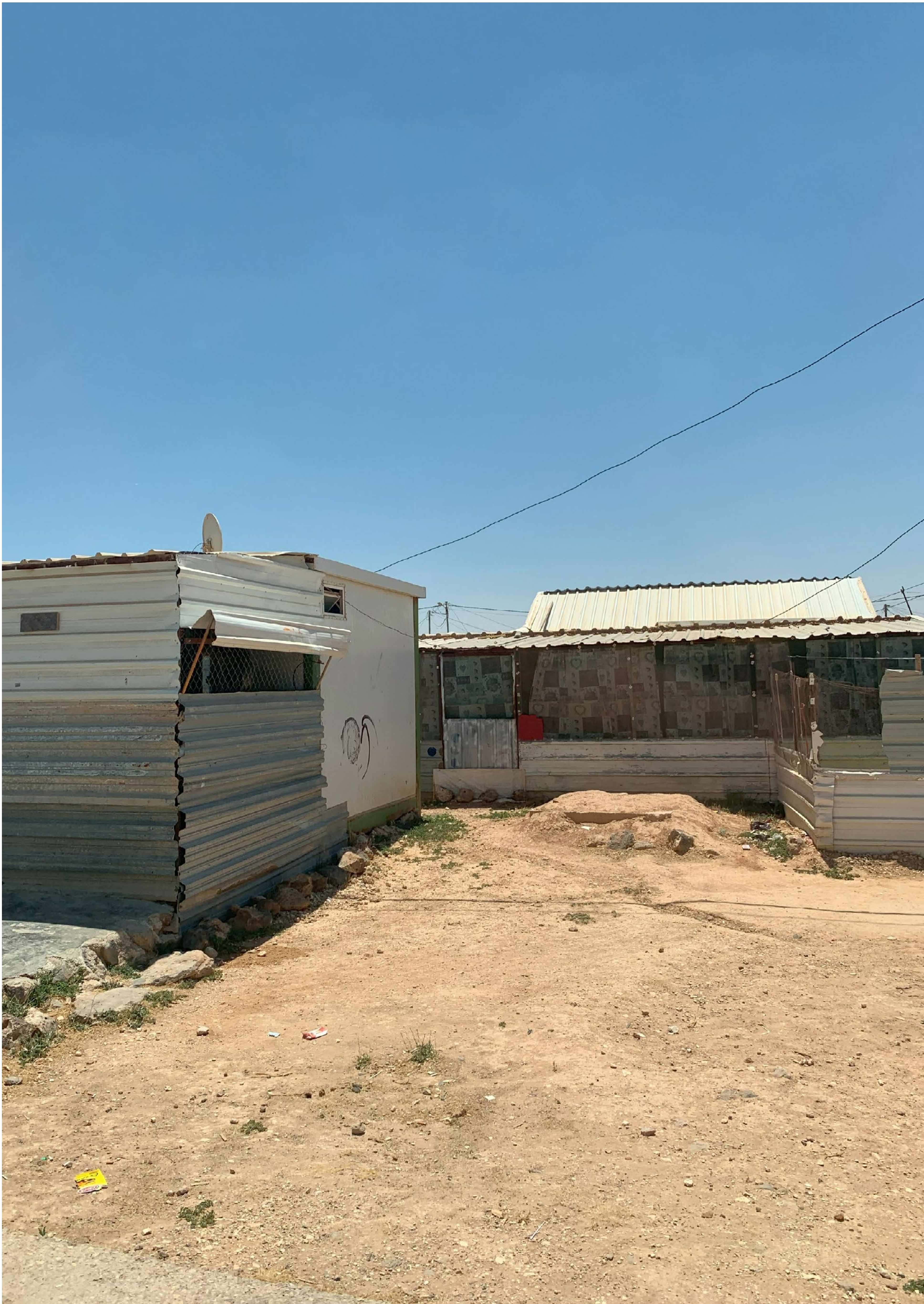
Figure 08. Exterior of a residential cluster formed by combining multiple shelter units and modifying them to meet residents' needs.
