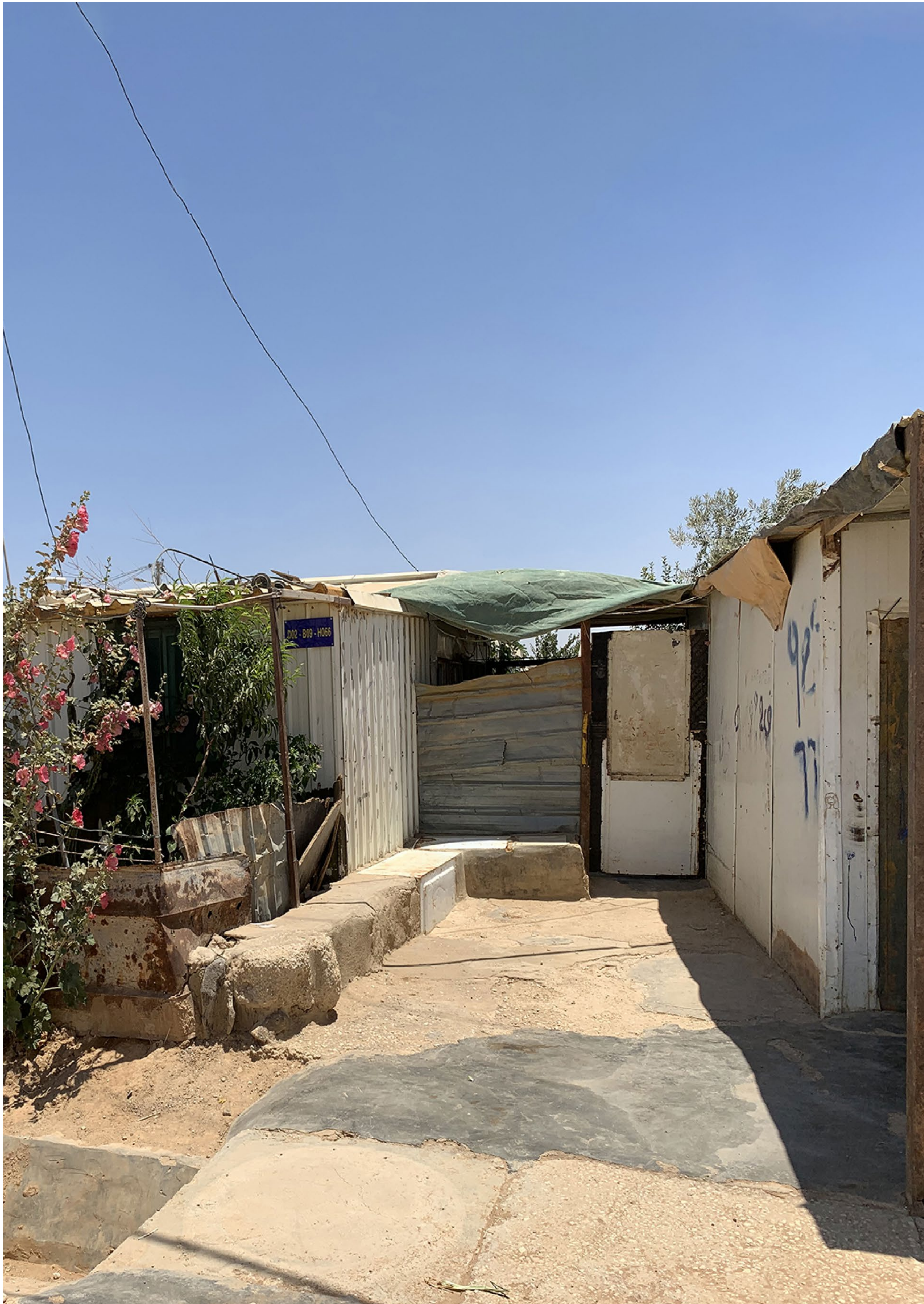
Figure 10. Exterior of a modified shelter cluster organised around a shared courtyard that functions as both a social space and a climatic buffer.
