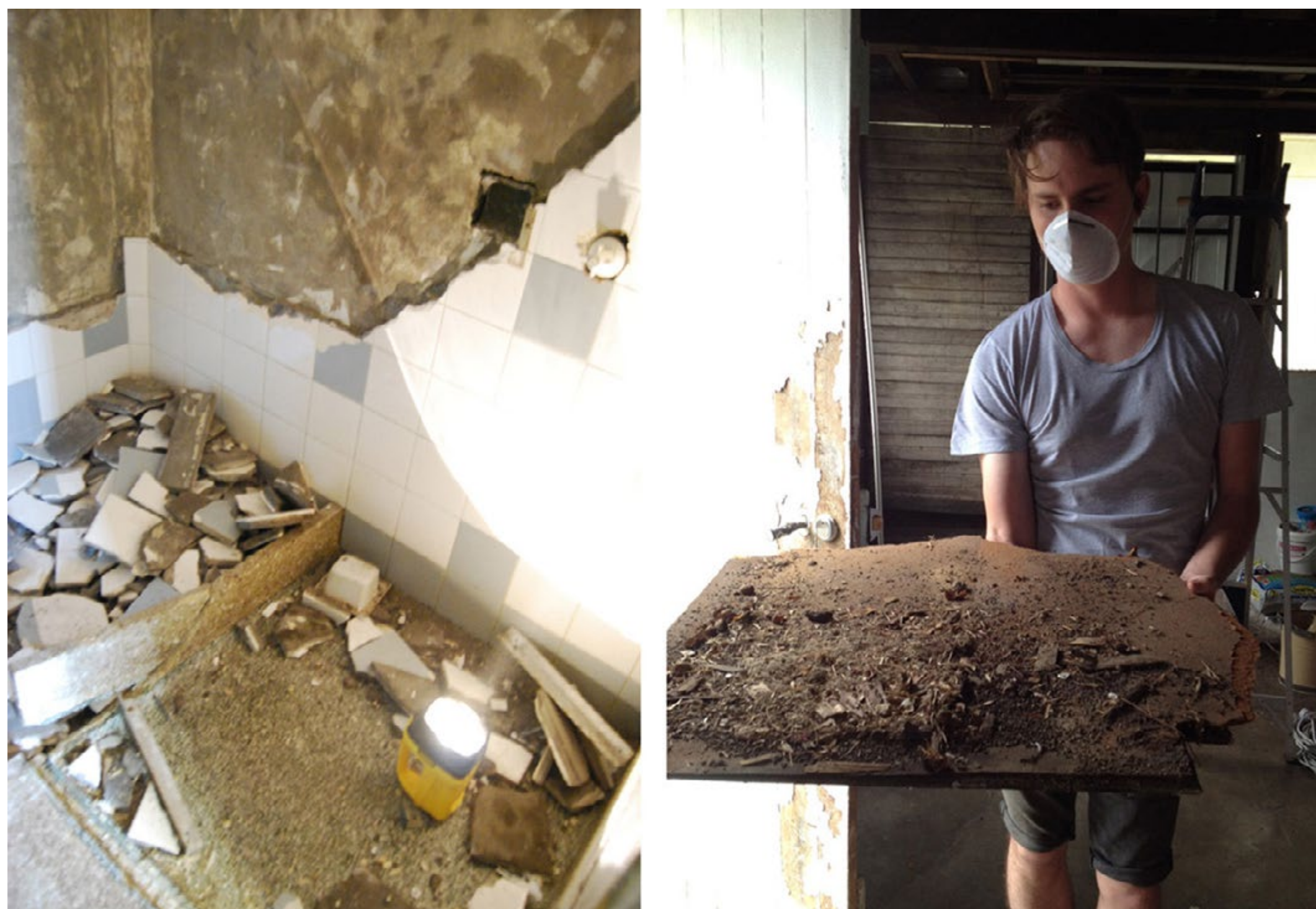
Figure 11. Demolition material and detritus, 2011. Photograph: Zuzana Kovar.
