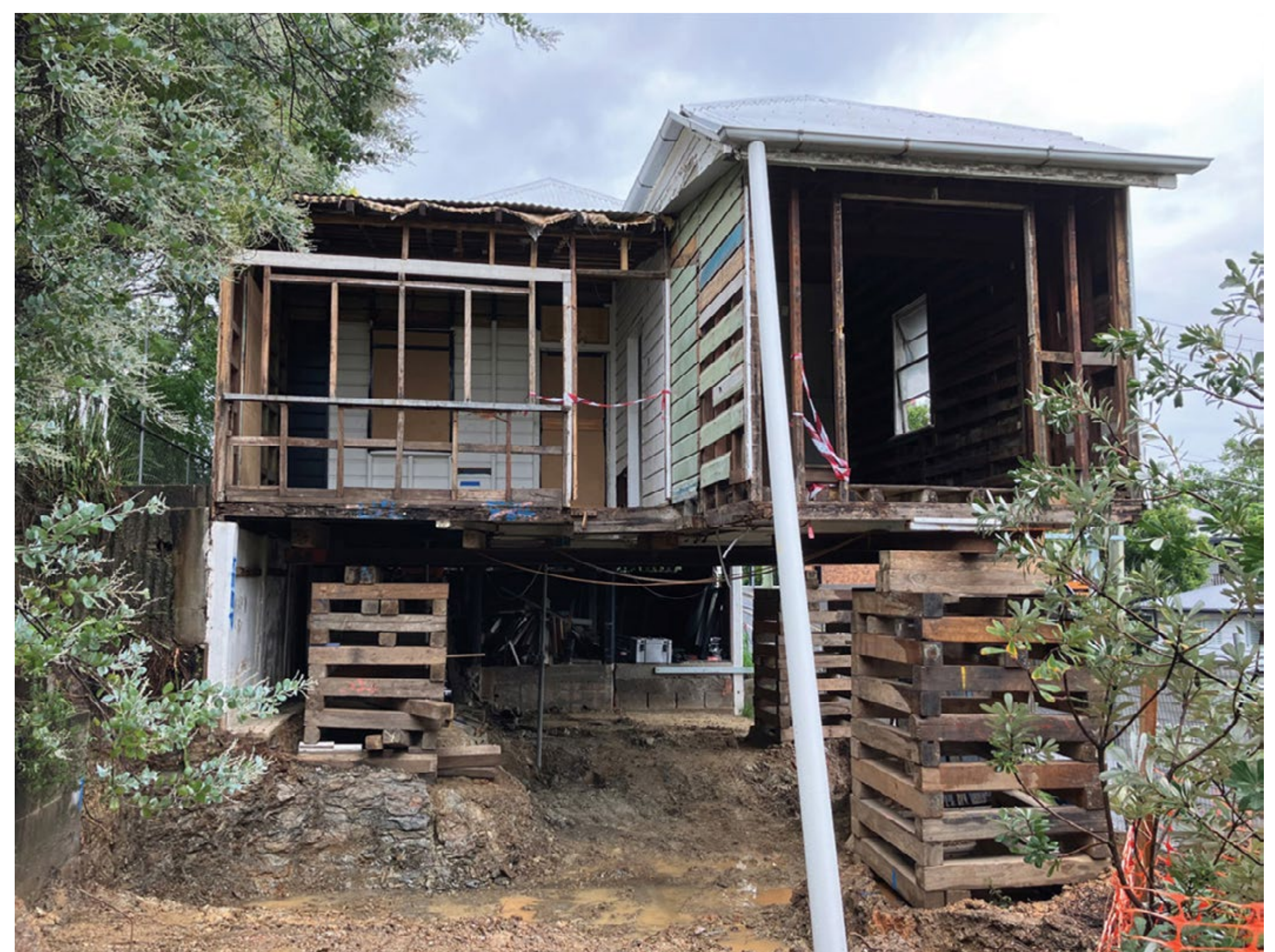
Figure 02. House propped for renovation works, 2022. Photograph: Zuzana Kovar.
