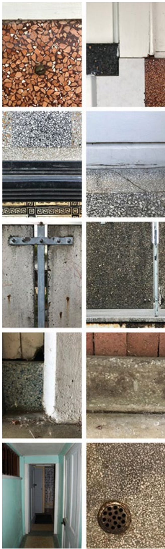
Figure 05. Terrazzo splashback, deck, balustrade, edging, floors, and shower tray. Photograph: Zuzana Kovar, 2011.
