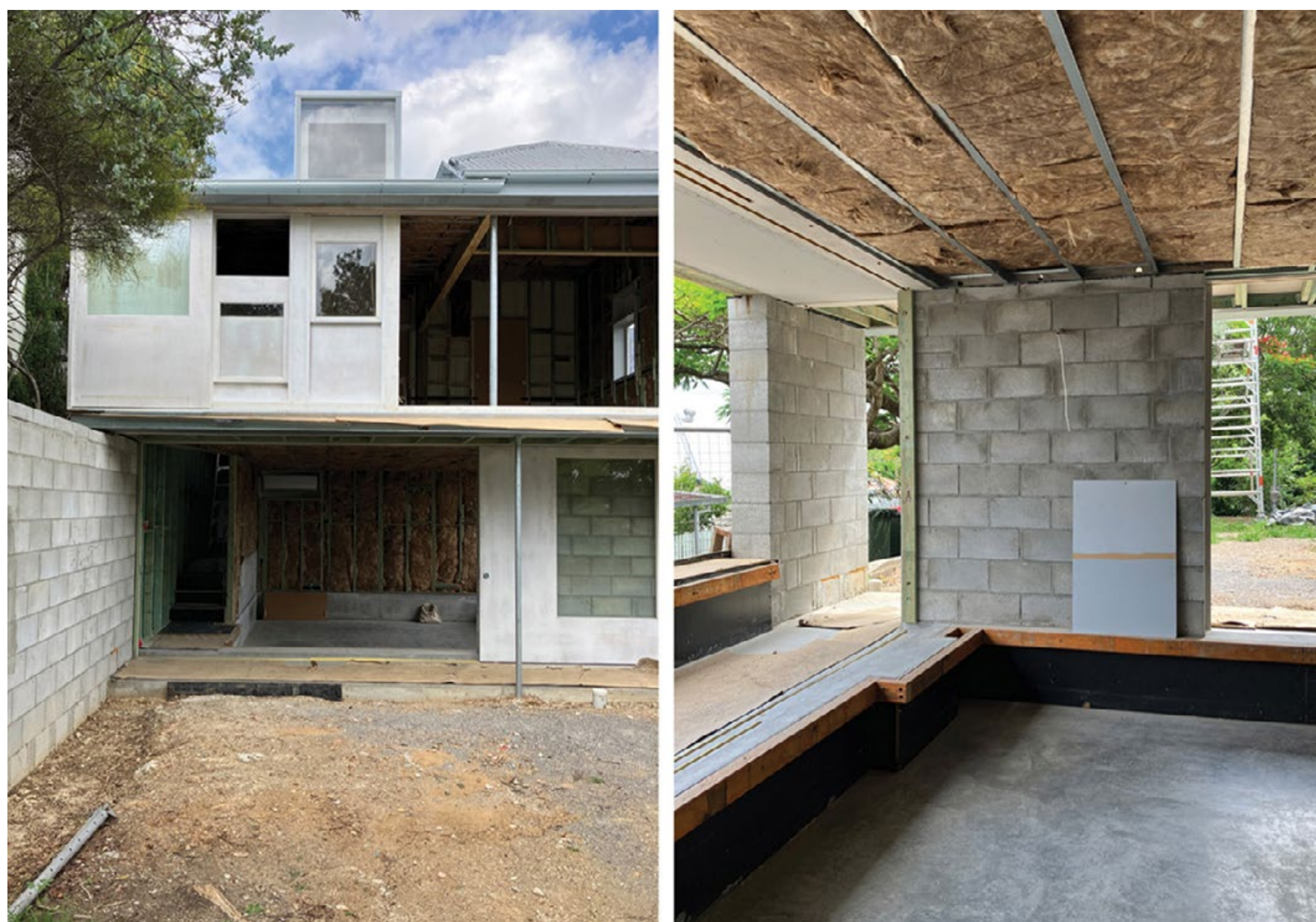
Figure 21. Rear elevation and studio with a view to the breezeway and garden. Photograph: Zuzana Kovar, 2022.
