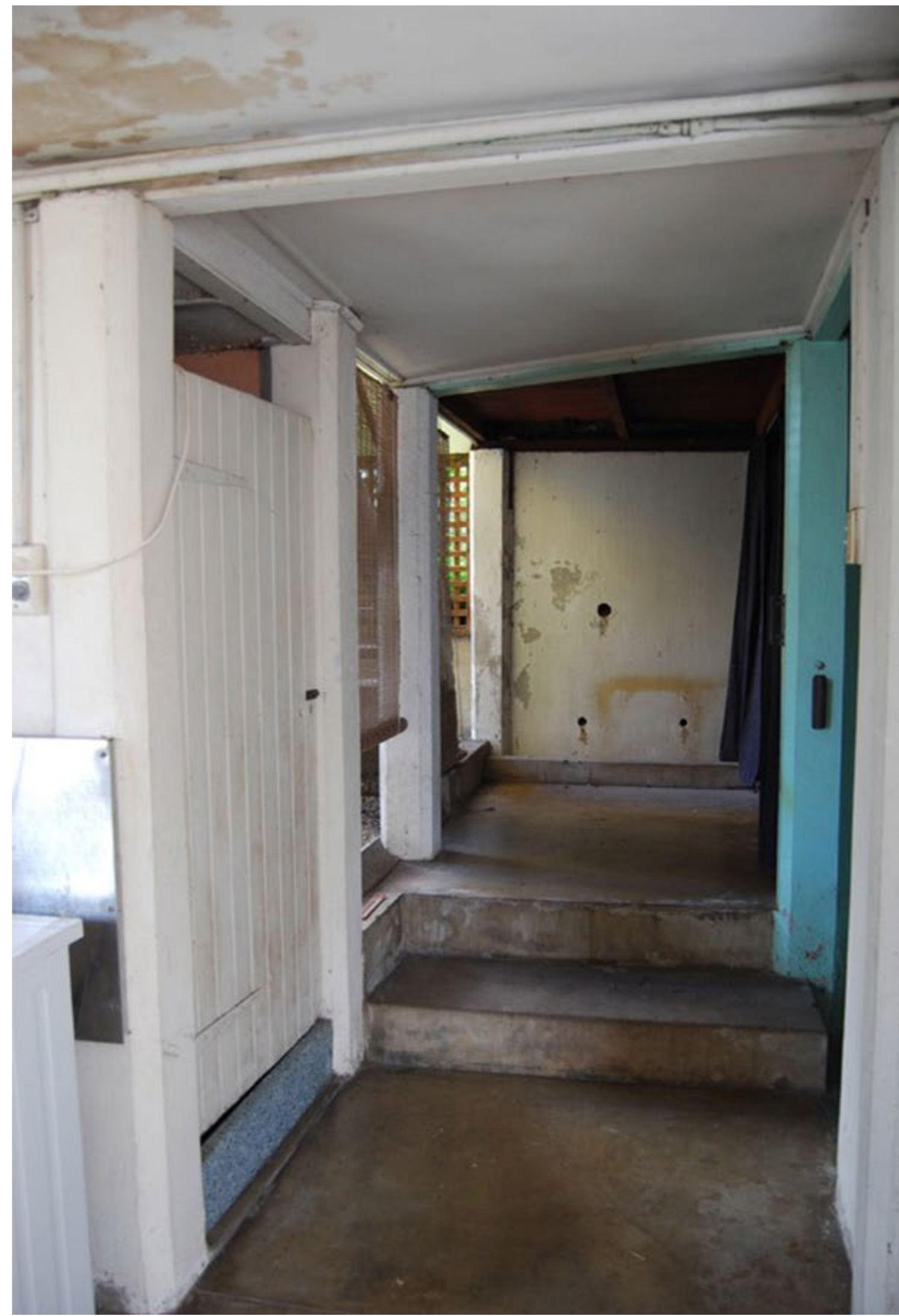
Figure 06. Concrete understorey. Photograph: Zuzana Kovar, 2011.
