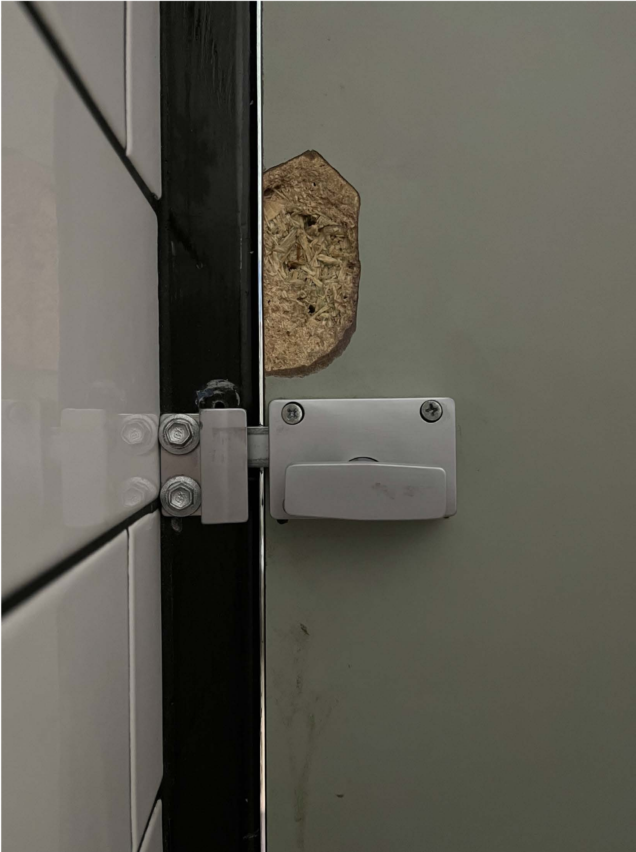
Figure 04. Toilet cubicle Melbourne, 2023. Image taken by author.
