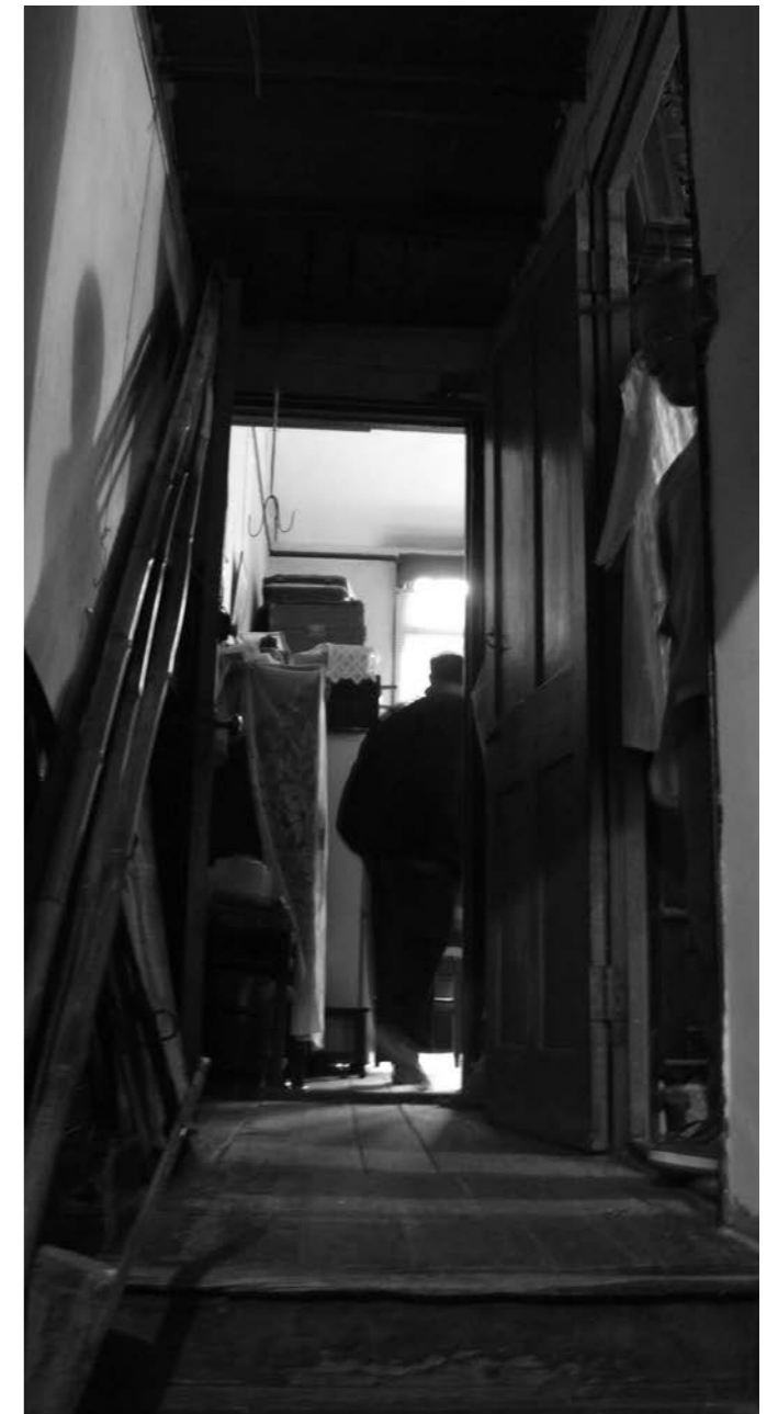
Above left Figure 5: Steep stairs before reconstruction. All photographs taken by the authors unless further indicated. Above right Figure 6: Chaotic interior.
