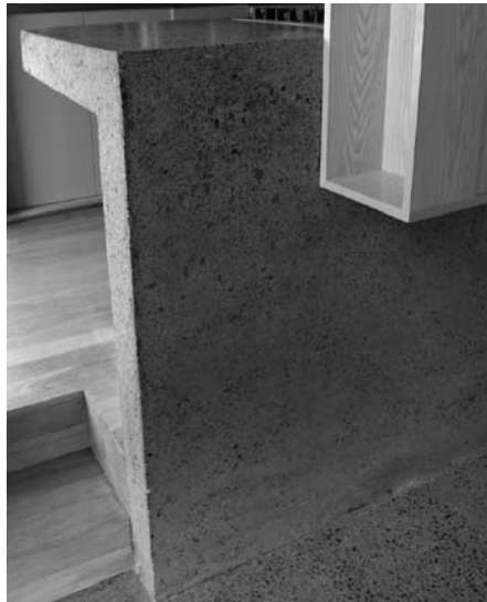
Figure 2: Folded concrete slab.
