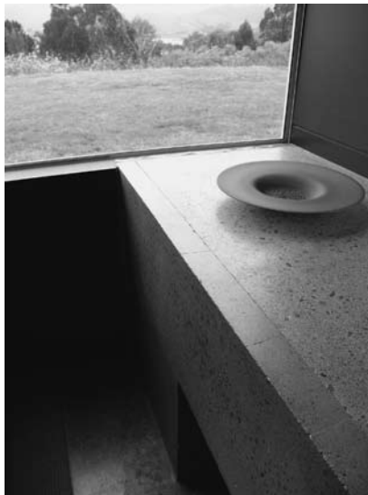
Figure 1: Ground level concrete slab
