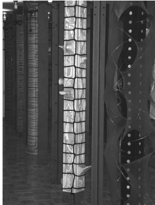
Figure 3: Column cladding photo (Photography: Author)
