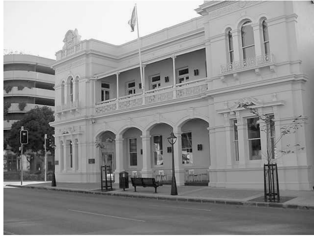
Figure 1: External view of main section of the refurbished post office (Photography: Author)
