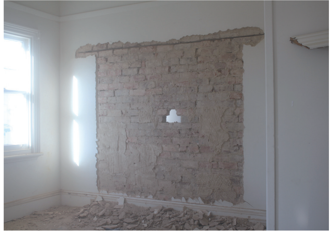
Prahran House. 2011. House. Two days. Locating. Drawing. Removal. Cutting. Removal.
