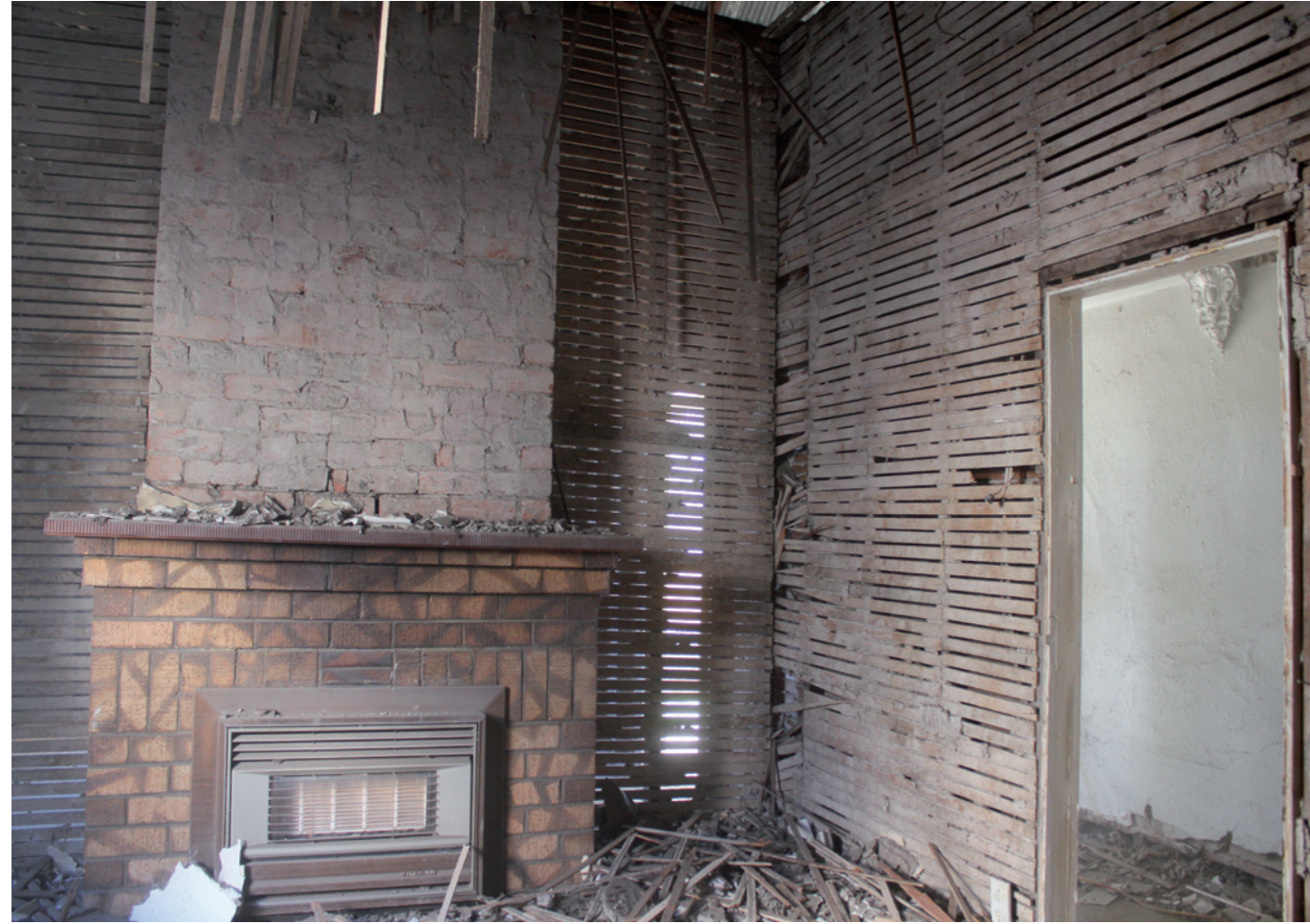
Critchley House. 2011. House. Two days. Locating. Removal. Removal. Removal.
